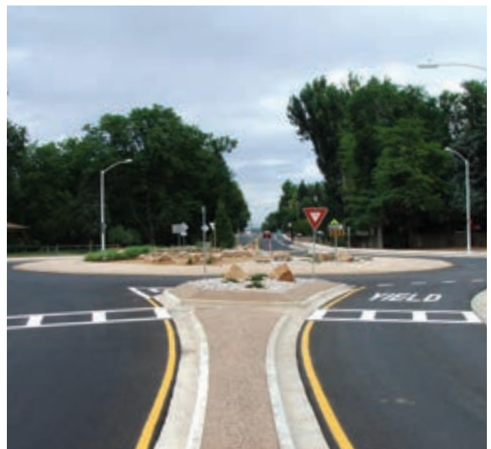
Roundabout with Mountable Apron
