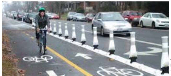
Raised Channelizing Systems using Qwick Kurb
