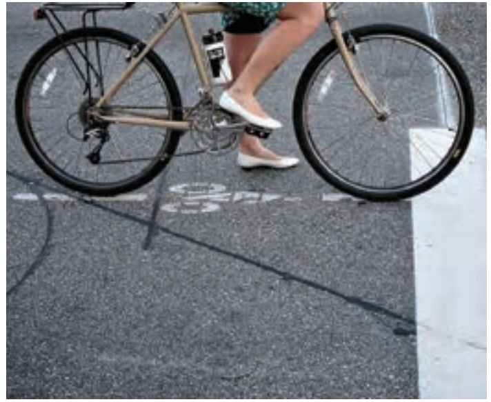
Pavement Markings Indicate the Bicycle Signal Detection Location
