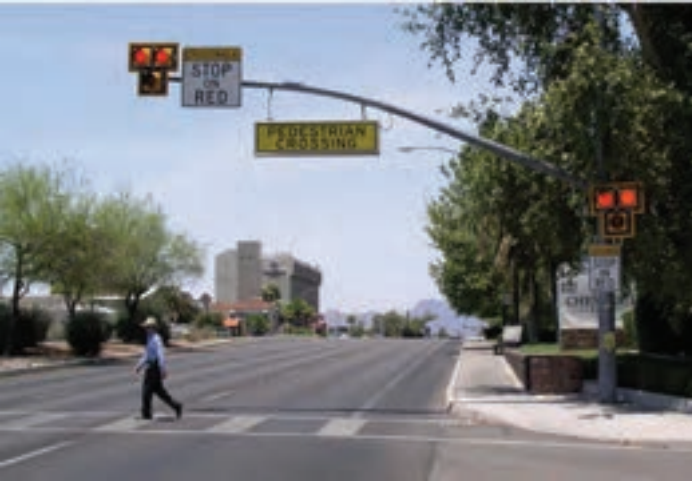
High-Intensity Activated crossWalk (HAWK)
